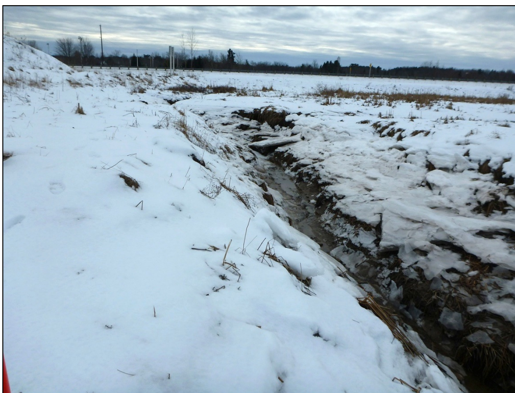
Figure 47 Excavated channel at SCE, 21 February 2014.
